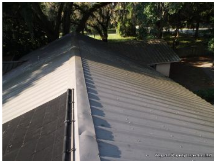
Appears serviceable. Walked entire roof.
